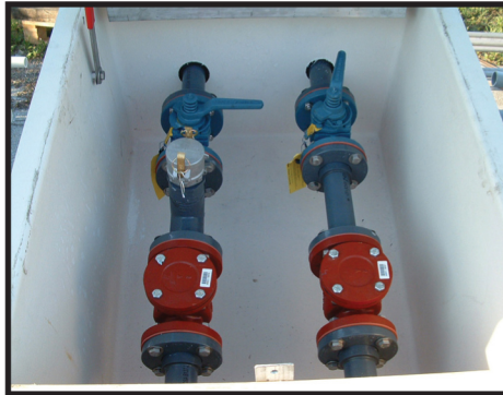
Standard Pump Valve Box 40"x30"x24" piped with SCH-80 PVC and flanged cast-iron Check and Plug Valves.
